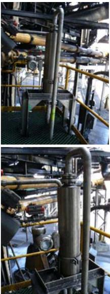
**Caption: OPTIMASS 7300 installed in tailings thickener underflow line**
